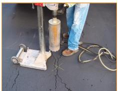
Deflection and core testing, when combined, provide data that is essential for designing structurally sound, long-lasting pavement at the lowest cost.
